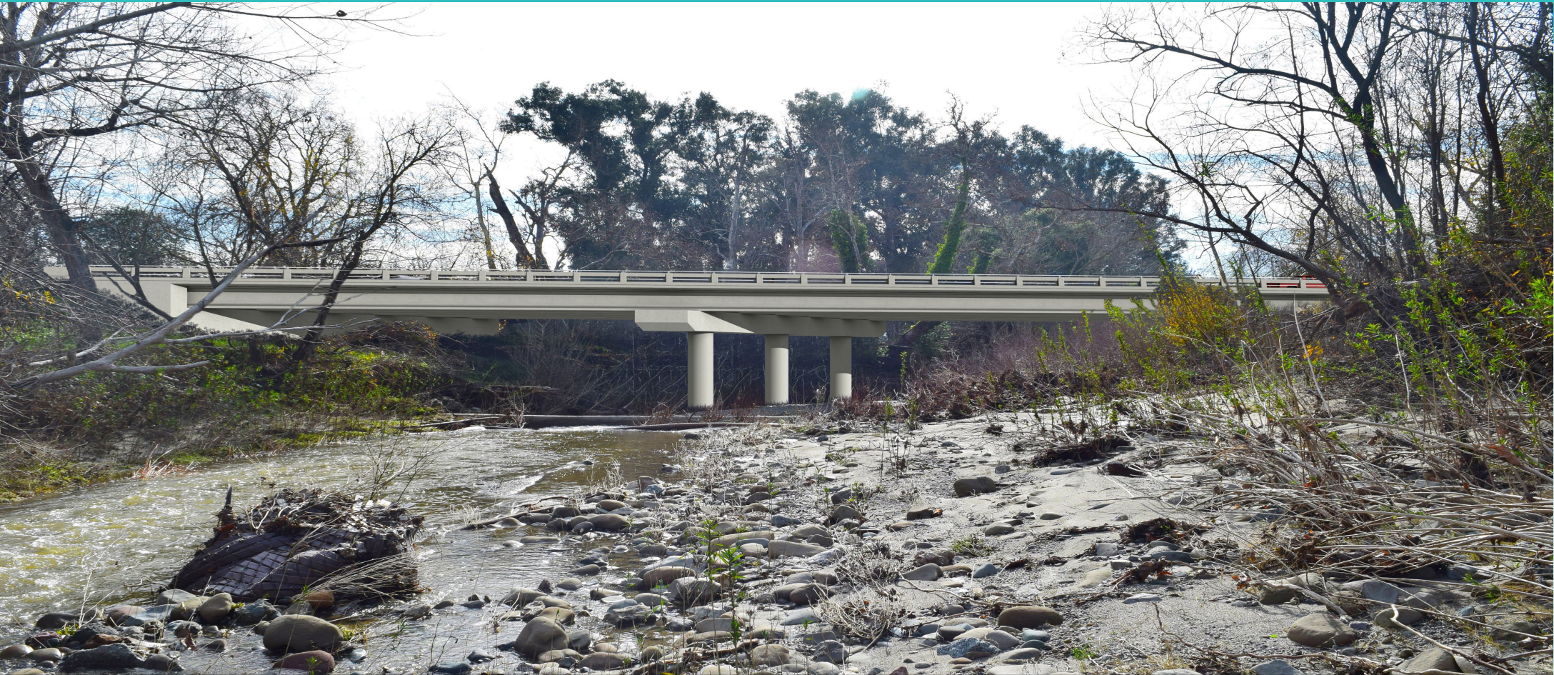
ARROYO DE LA LAGUNA CREEK BRIDGE STATE ROUTE 84, ALAMEDA COUNTY, CALIFORNIA VIEW 1 - PROPOSED BRIDGE
