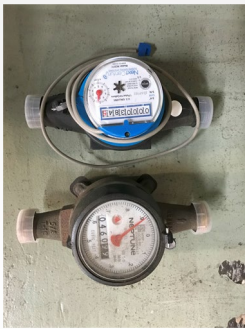
Figure 5 Examples of water submeters commonly used in multifamily residences.
