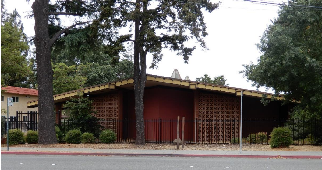
20055 Redwood Road, Castro Valley, east façade, view west (ARG, July 2021)
