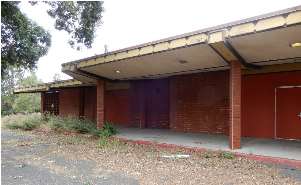
Figure 2. South façade, west portion, view northwest (ARG, July 2021)
