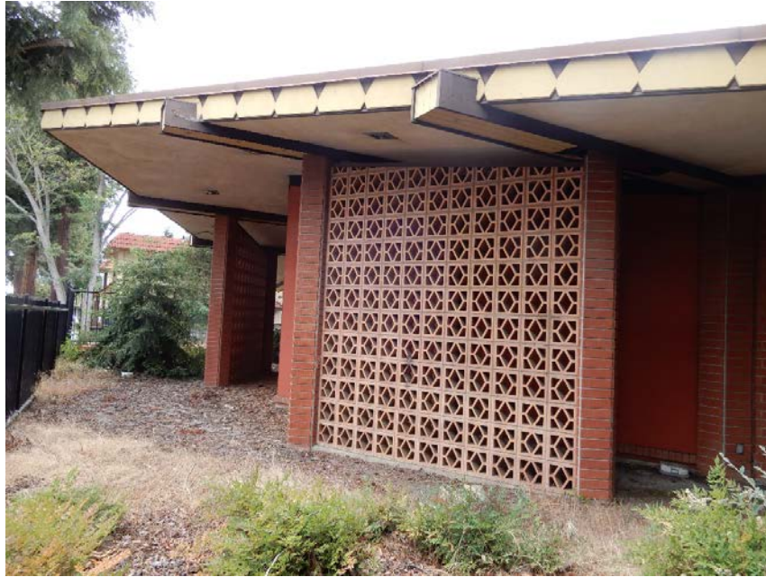
Figure 5. East façade, north portion, view southwest (ARG, July 2021)
