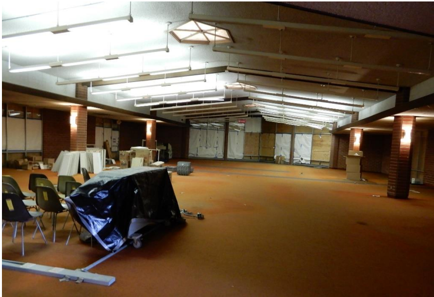
Open plan area at east side, view east (ARG, July 2021)
