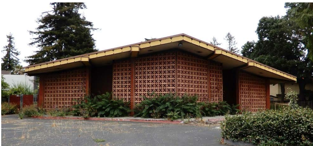
Figure 6. West façade, view east (ARG, July 2021)
