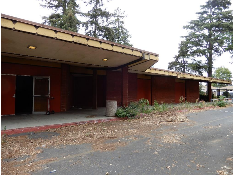
South façade, east side, view northeast (ARG, July 2021)
