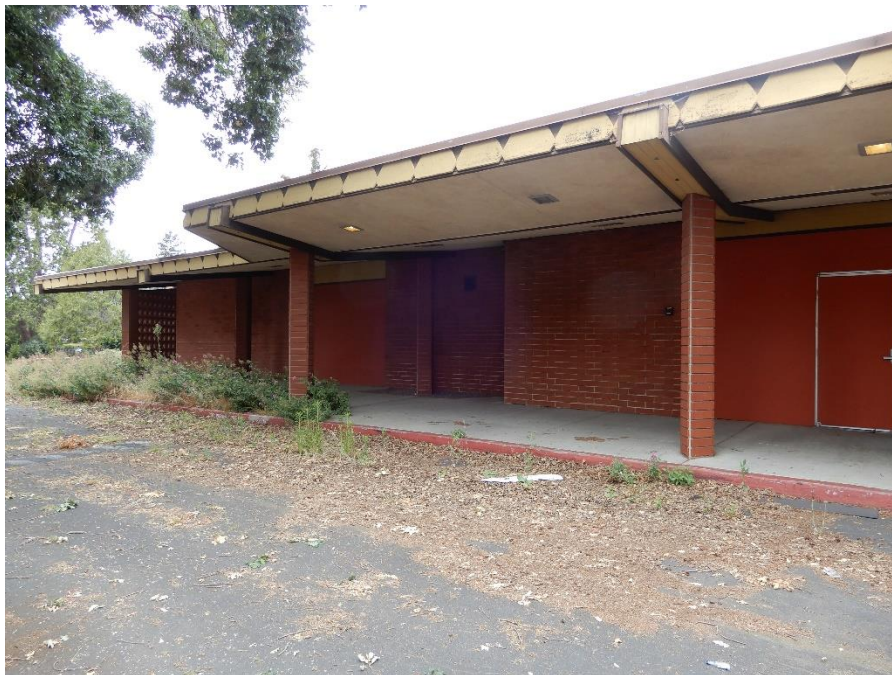
South façade, west side, view northwest (ARG, July 2021)
