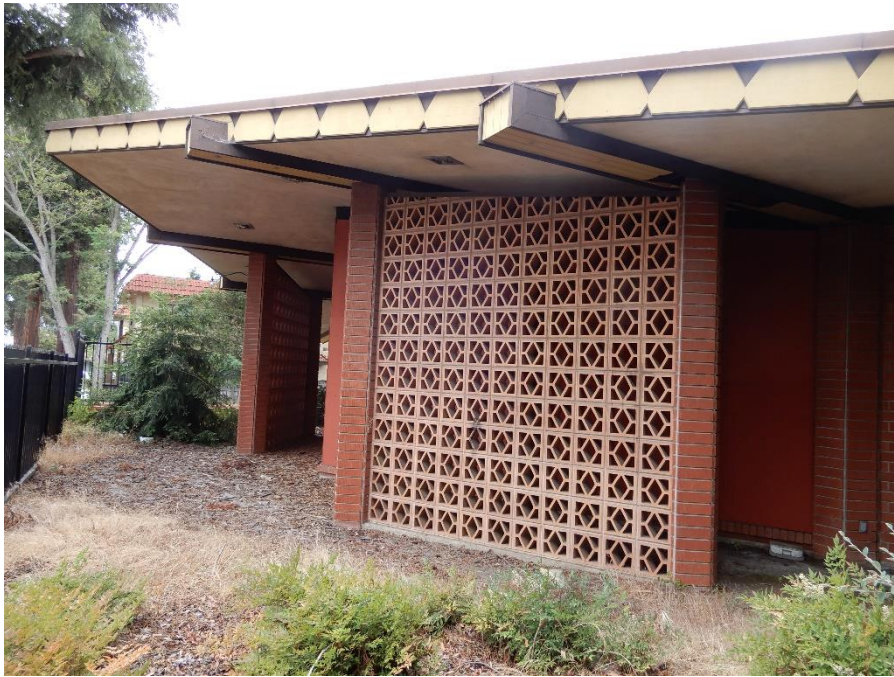
East façade, north side, detail of breeze block, view southwest (ARG, July 2021)
