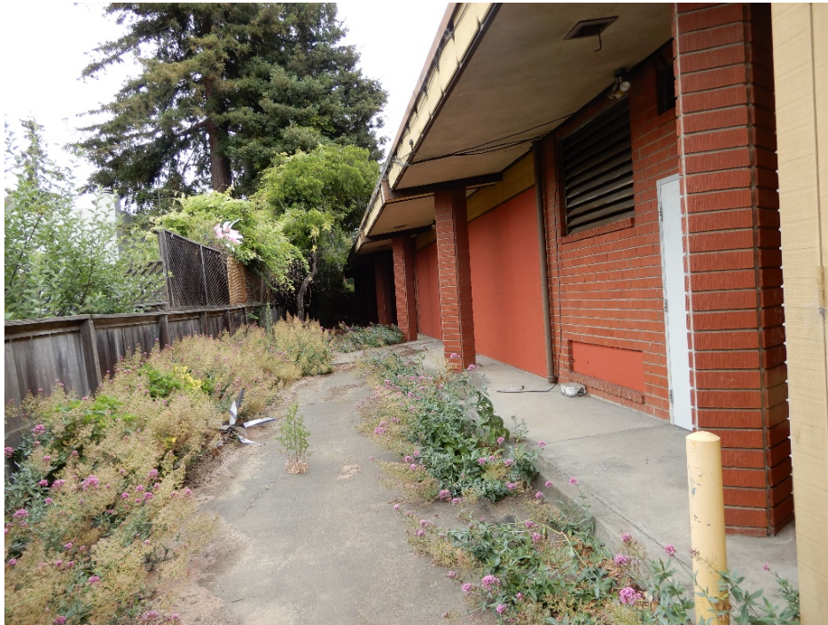
Figure 7. North façade, view east (ARG, July 2021)
