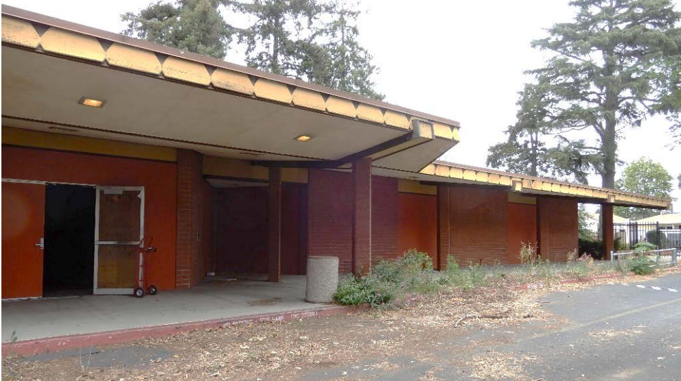
Figure 3. South façade, east portion, view northeast (ARG, July 2021)
