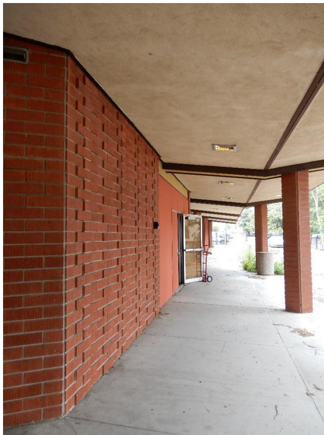
South façade, detail of brick and columns, view east (ARG, July 2021)
