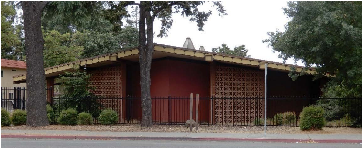
Figure 1. 20055 Redwood Road, Castro Valley, east façade, view west (ARG, July 2021)
