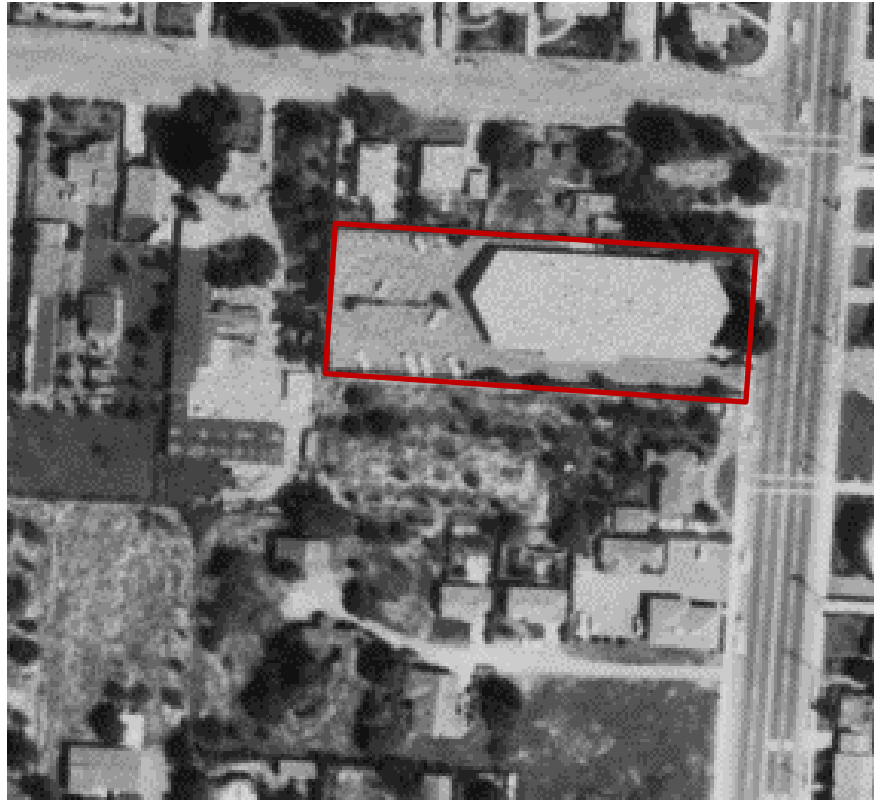
Figure 13. 1965 aerial photograph, site of the subject property lot outlined in red (UCSB FrameFinder, cas-65-130_5-39)
