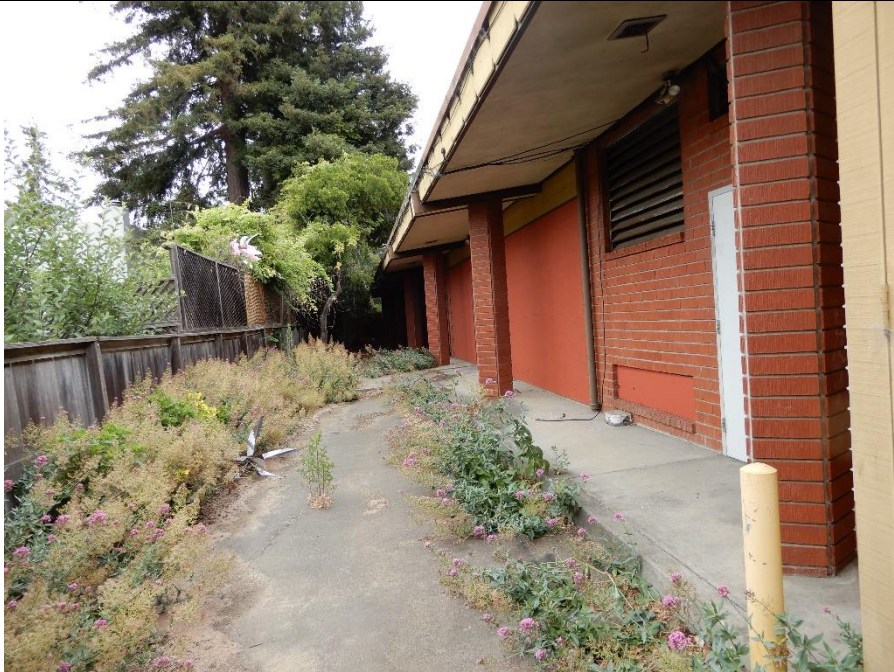
North façade, view east (ARG, July 2021)
