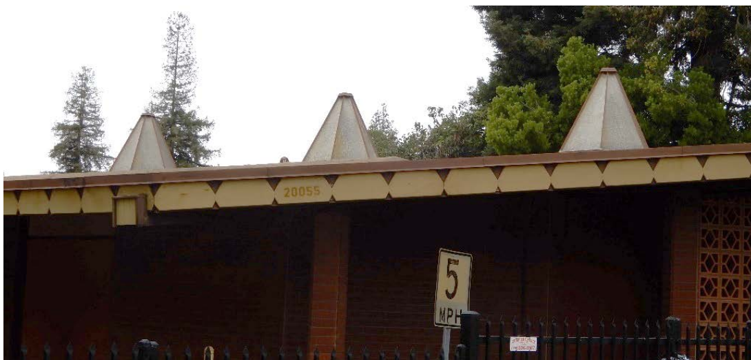
Figure 8. Skylights, view northwest (ARG, July 2021)
