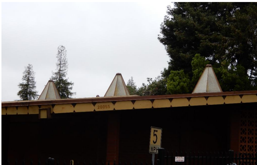
Roofline showing skylights, view northwest (ARG, July 2021)
