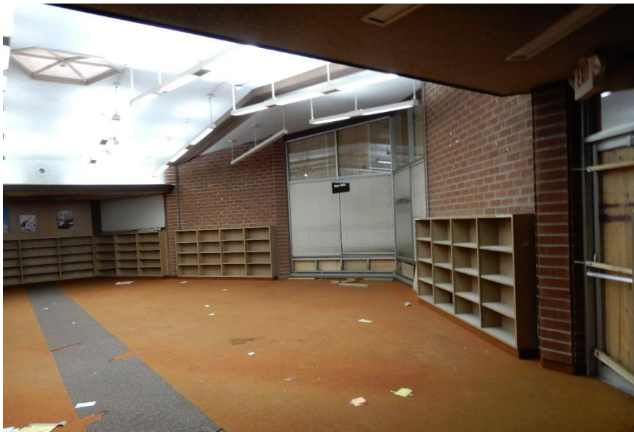
Open plan area at west side, view southwest (ARG, July 2021)
