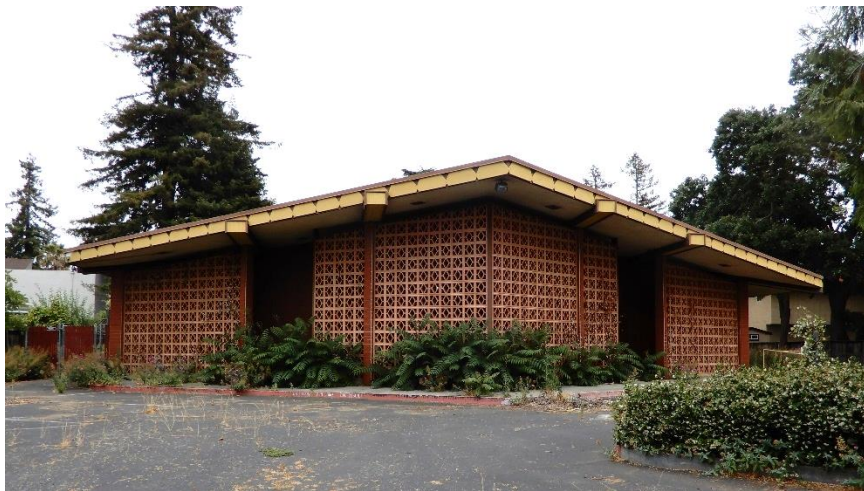
West façade, view east (ARG, July 2021)
