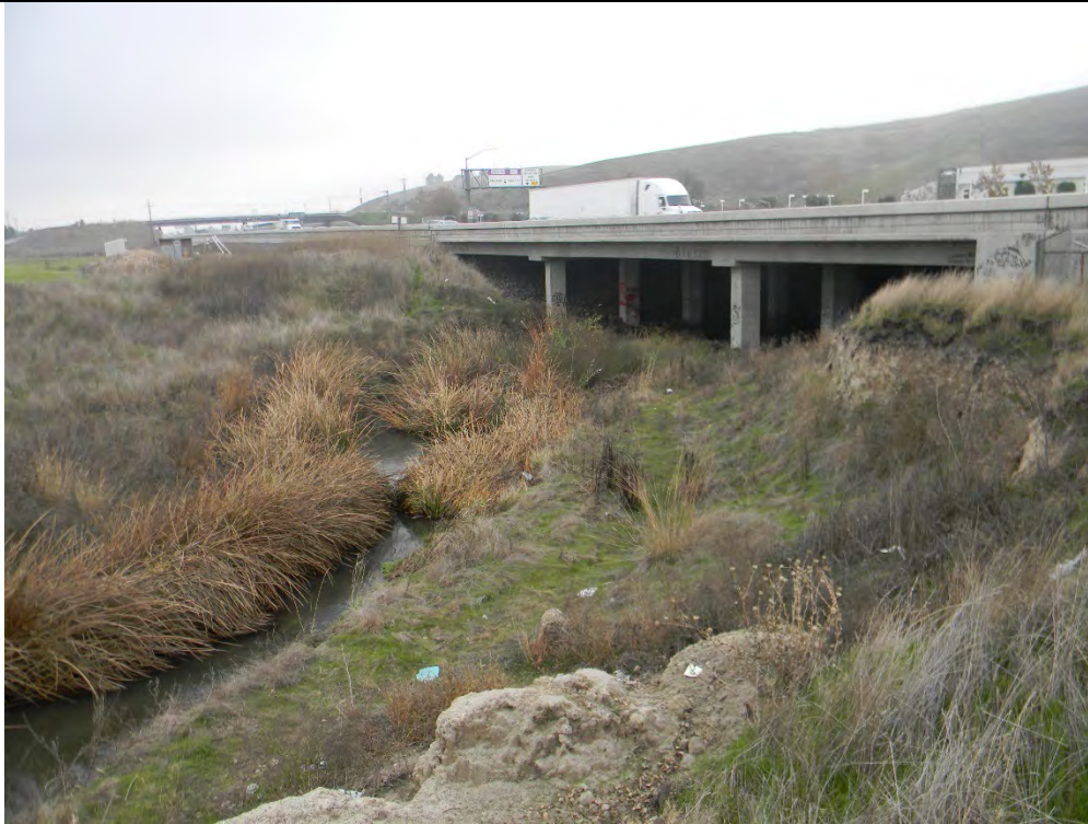
6. Photograph from the northwest of Arroyo Las Positas flowing underneath Arthur H Breed, Jr Freeway
