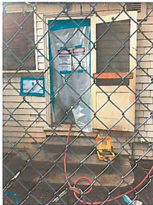
Photo 2 – Entry to containment
