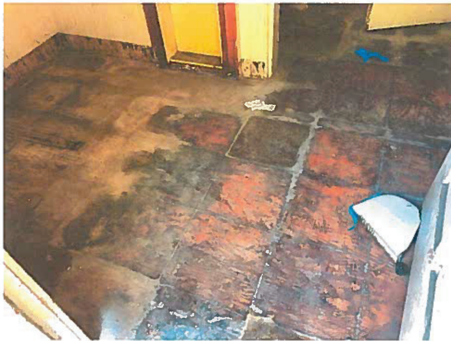
Photo 7 – Laundry Room post-abatement
