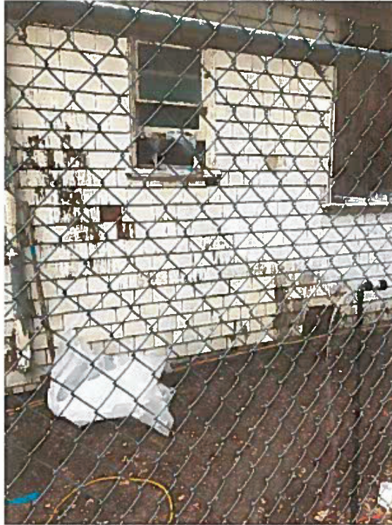
Photo 3 – Containment exhaust port
