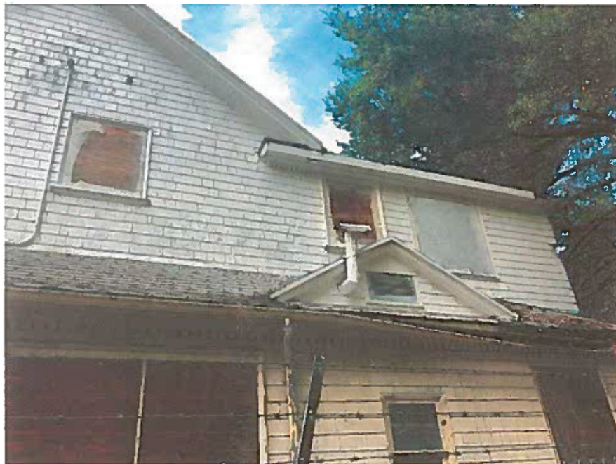
Photo 18 – Paint work on second story
