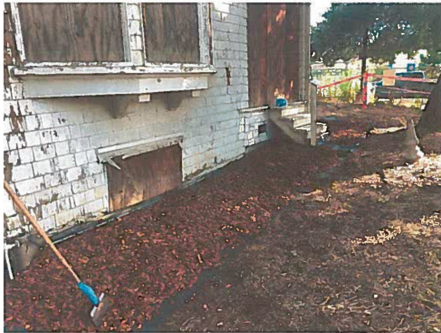
Photo 19 – In process of laying woodchips and fabric barrier
