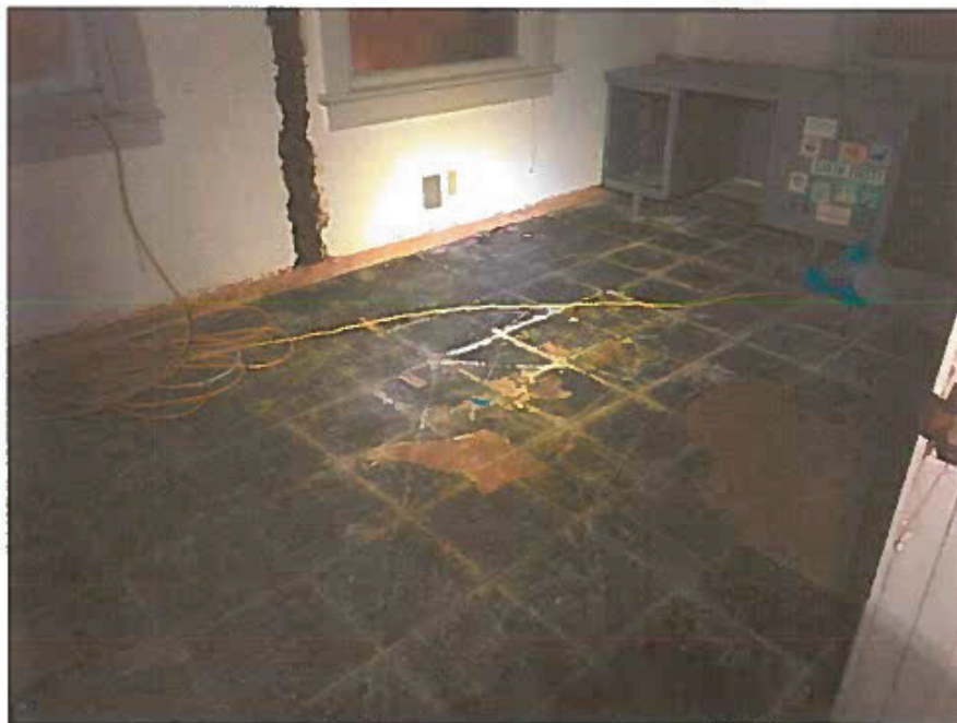
Photo 14 – Northeast Room post-abatement
