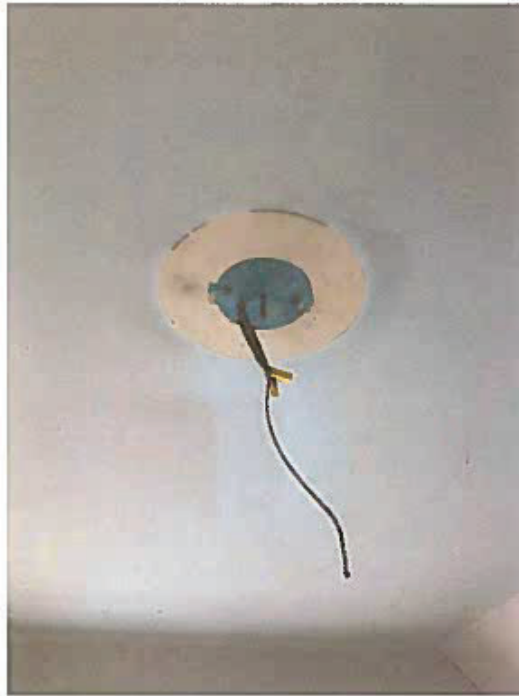
Photo 15 – Light fixture post-abatement
