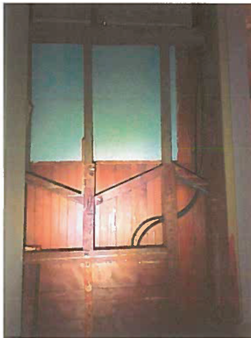
Photo 10 – Fireplace Hallway post-abatement
