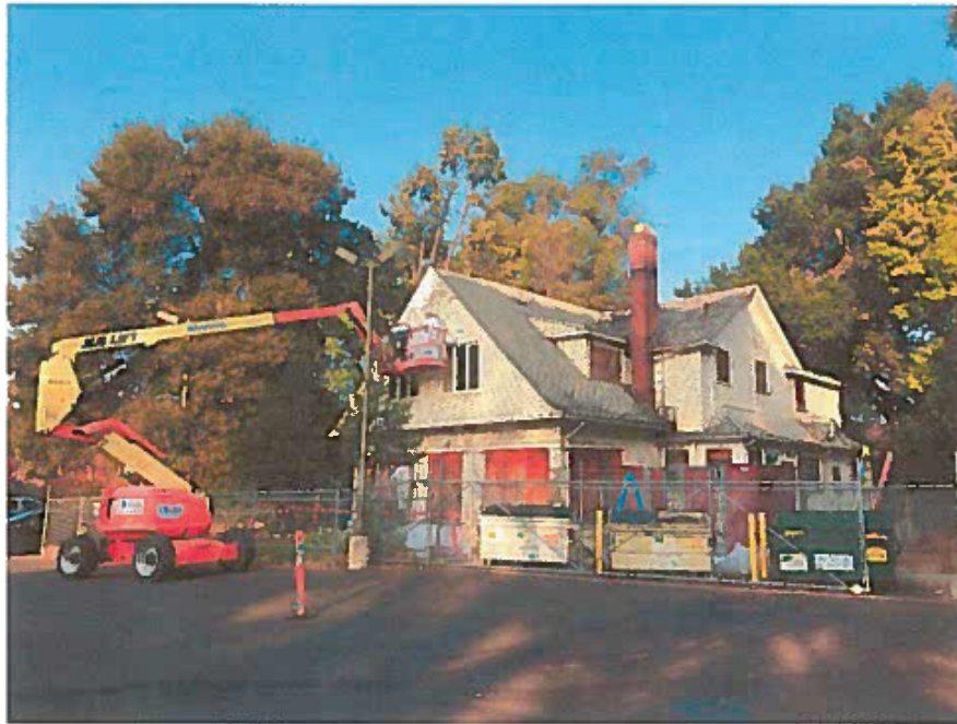
Photo 1 – Using telescopic manlift to scrape upper section of White Cotton Cottage
