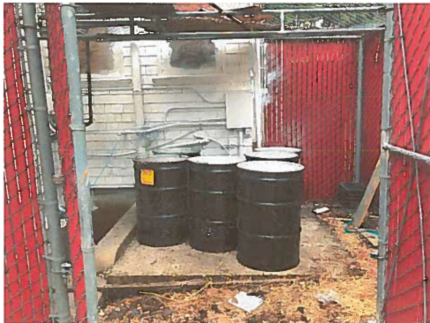
Photo 20 – Lead drums staged in locked area
