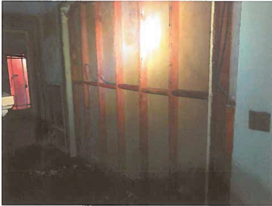
Photo 9 – Fireplace Hallway post-abatement
