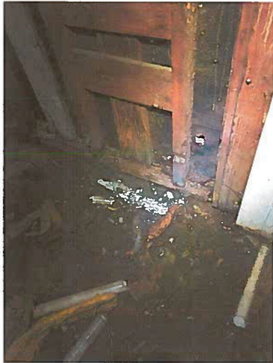
Photo 6 – Removal of 2 feet of pipe insulation: Basement
