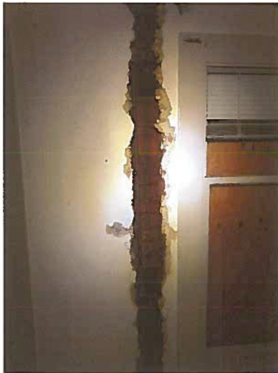
Photo 4 – Removal of 12 feet of radiator pipe insulation: first story
