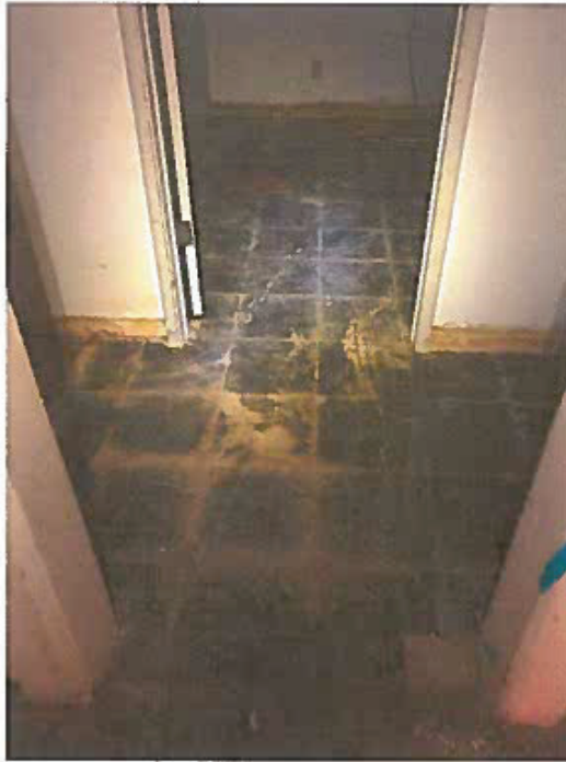
Photo 13 – Hallway leading to Northeast Room post-abatement
