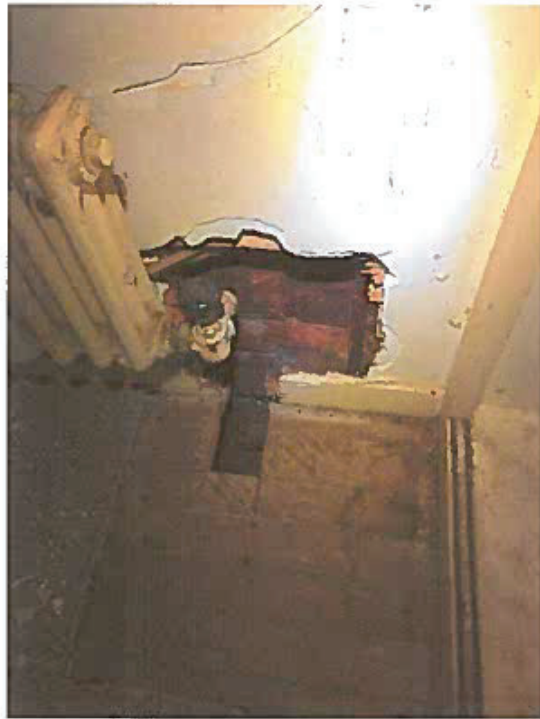
Photo 5 – Removal of 12 feet of radiator pipe insulation: second story
