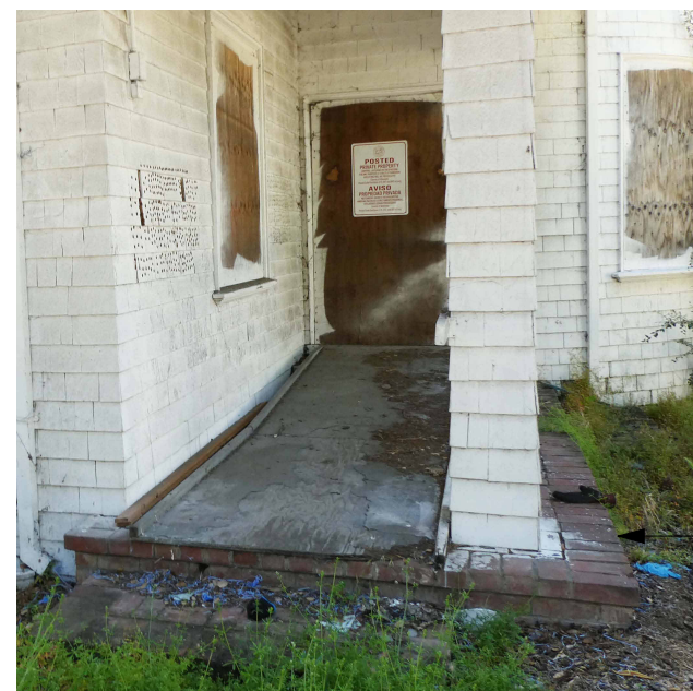
S11 - BRICK MASONRY AT PORCH
