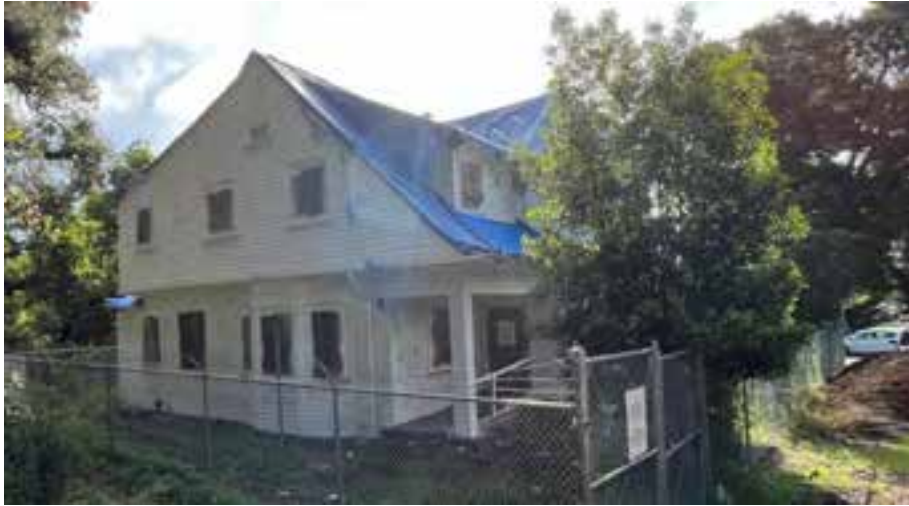
Figure 4. North elevation, west end.
