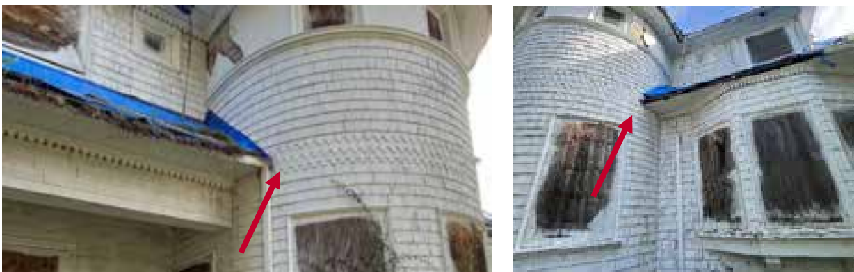
Figures 13 and 14. West elevation, tower, looking south (left) and looking north (right). Change in shingles from square butt to diamond and L-shaped identified with red arrows.
