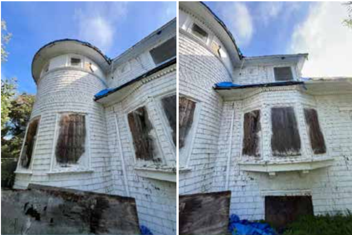
Figures 11 and 12. Detail of the rounded tower (left) and the bay window (right) on the west elevation.
