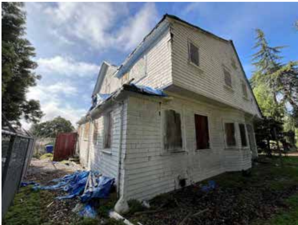
Figure 3. North elevation, east end.
