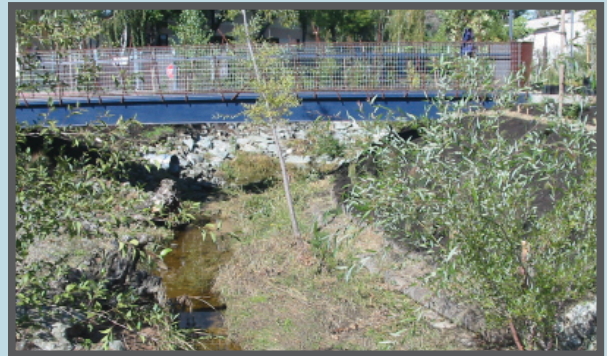
Pedestrian bridge over newly restored Castro Valley Creek.
