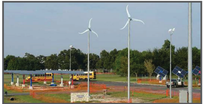
The Santa Rita Jail Smart Grid includes small wind turbines, advanced battery energy storage, and solar hot water.
