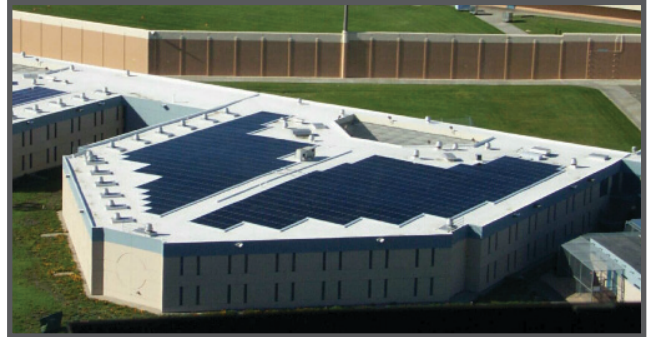
EPA recognized Alameda County for on-site solar power, including this 1.18 megawatt installation at Santa Rita Jail.
